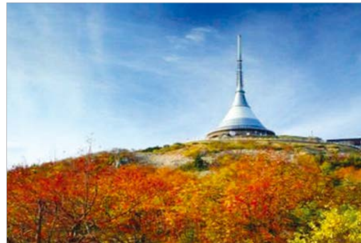
Fig. 21: The transmission tower on Ještěd; a constructed natural landmark
