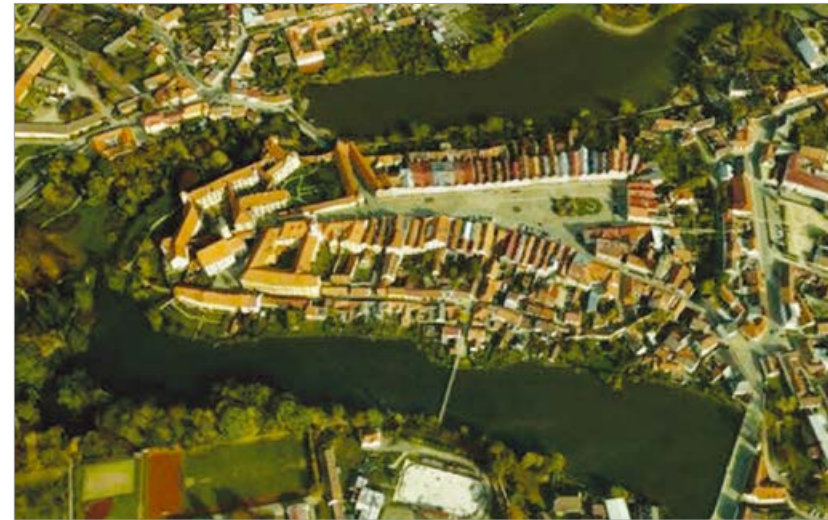
Fig. 17: Aerial photograph of the historic centre of Telč
