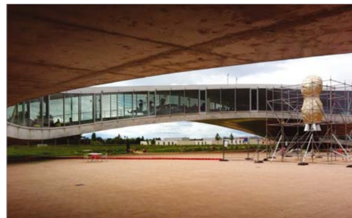
Fig. 36: A vista of surrounding landscape through a building, Lausanne
