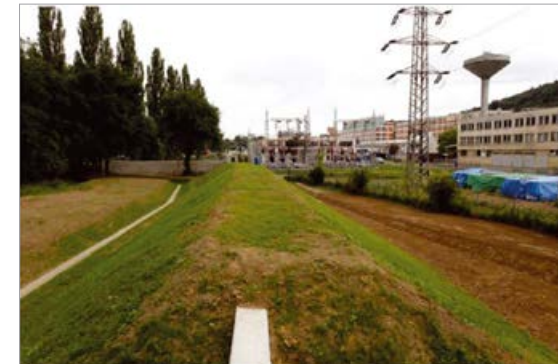
Natural resources Protective levees along a river, Napajedla References: http://www.cs-povodne.eu/
