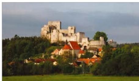
Fig. 45: Gradation of the mass of buildings, the Rabí Castle
